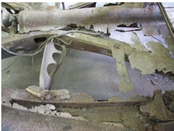
Fig. 4- LEFT What remained of the floor pan and a twisted frame cross-member
