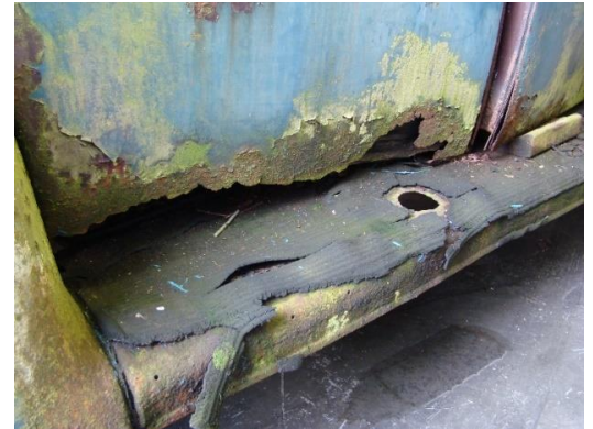
Fig. 1 - Quarter panel damage typical all around including doors
