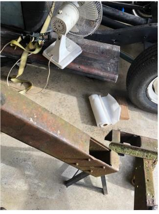
Here is the first section I cut out. Going from four stake pockets to three. I used a hack saw and took my time. I am too inaccurate with a cutting disc.
