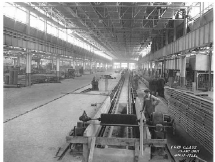
Glass plant under construction, 1925.
